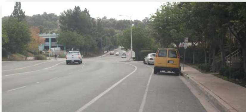
Class II Bike Lane along Market Street between 32 nd and I-15 SB Ramps.
